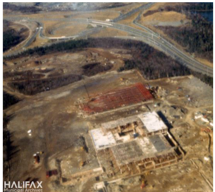
Mic Mac Mall Construction, 1972 (Halifax Municipal Archives)
