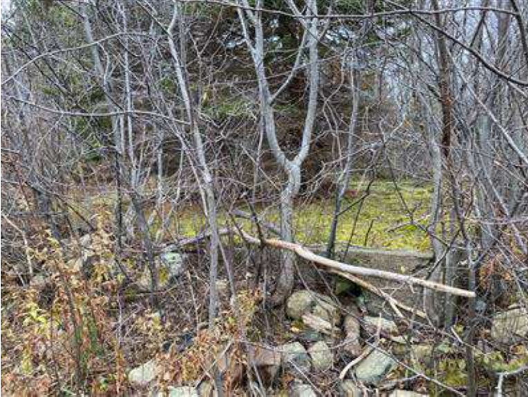
Photo 57 View northwest at MPR-ARCH-264 at a corner of a twentieth century foundation feature
