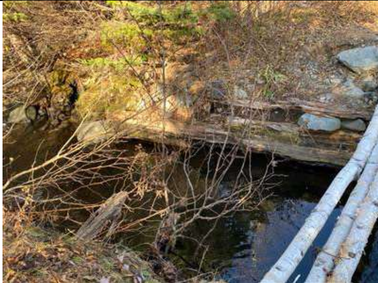
Photo 13 View east of an old bridge footing encountered along the northern section of the east branch of Smelt Brook at CKM-ARCH-164
