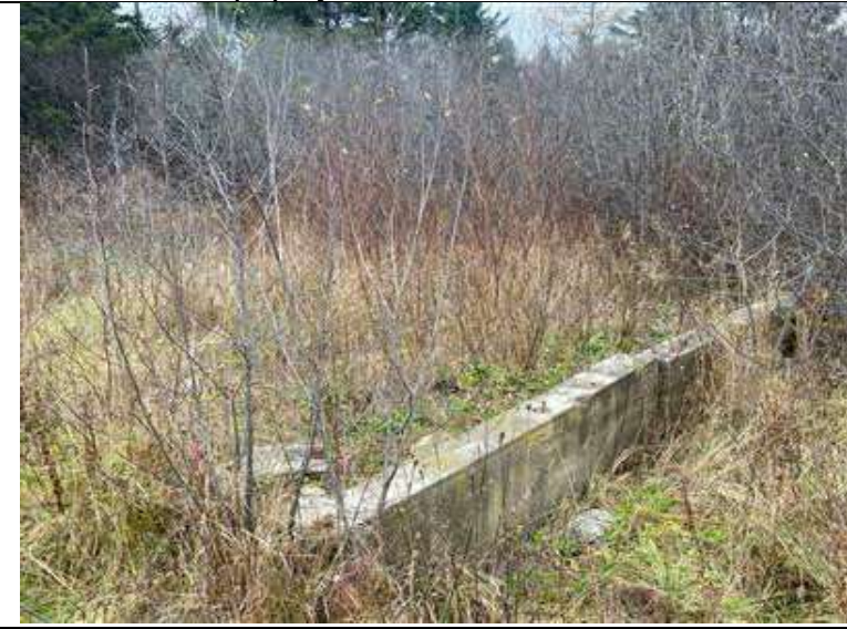
Photo 60 View southwest from JRK-HSF-014 at concrete foundation features associate with the Akoma property
