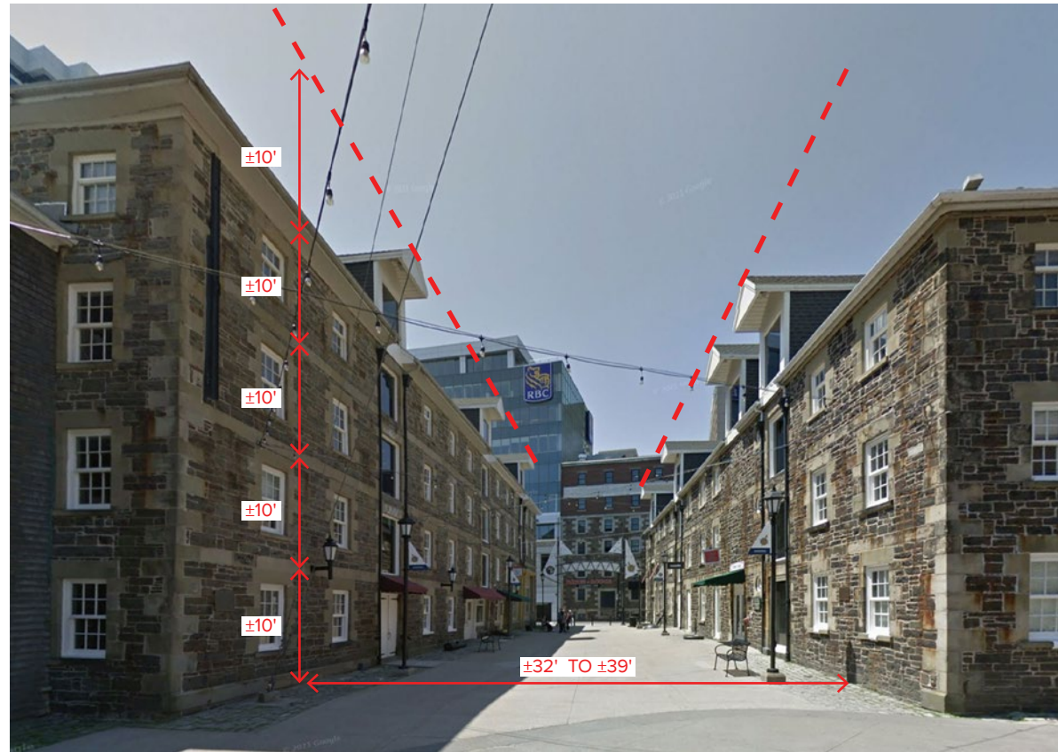
PRIVATEERS WHARF STREETSCAPE
