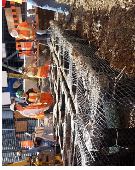
Example 3: Soil cells support healthy trees
