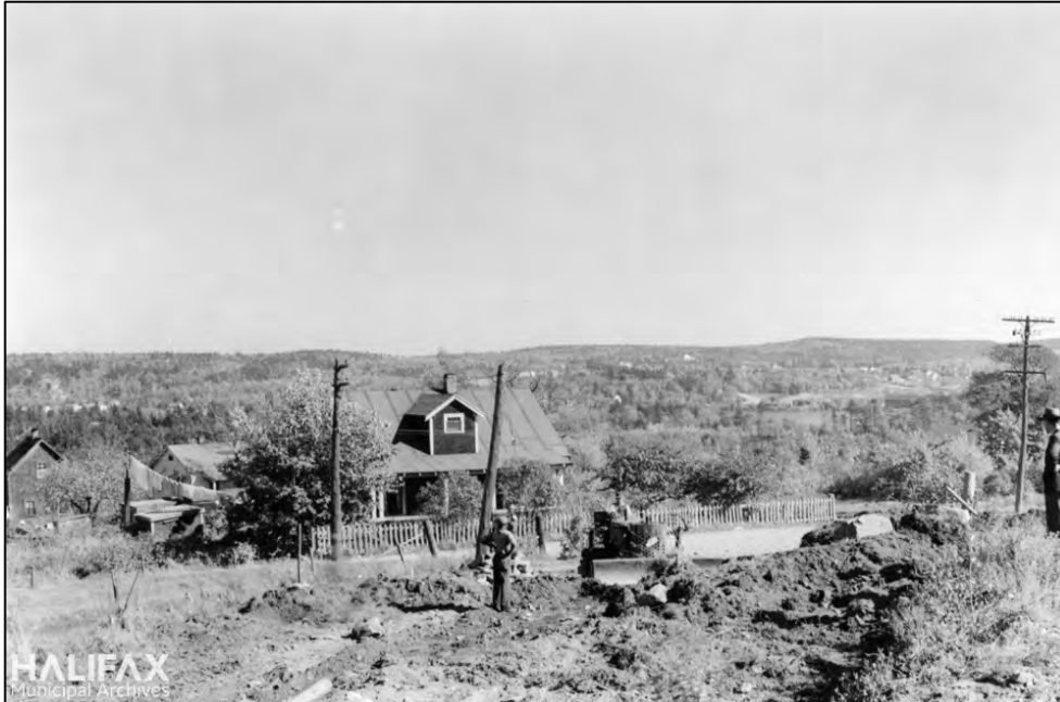
Figure 3.2-8: 238 Crichton Avenue, part of “the Avenue”, photographed in the 1940s during road work. 83 The house still stands today.
