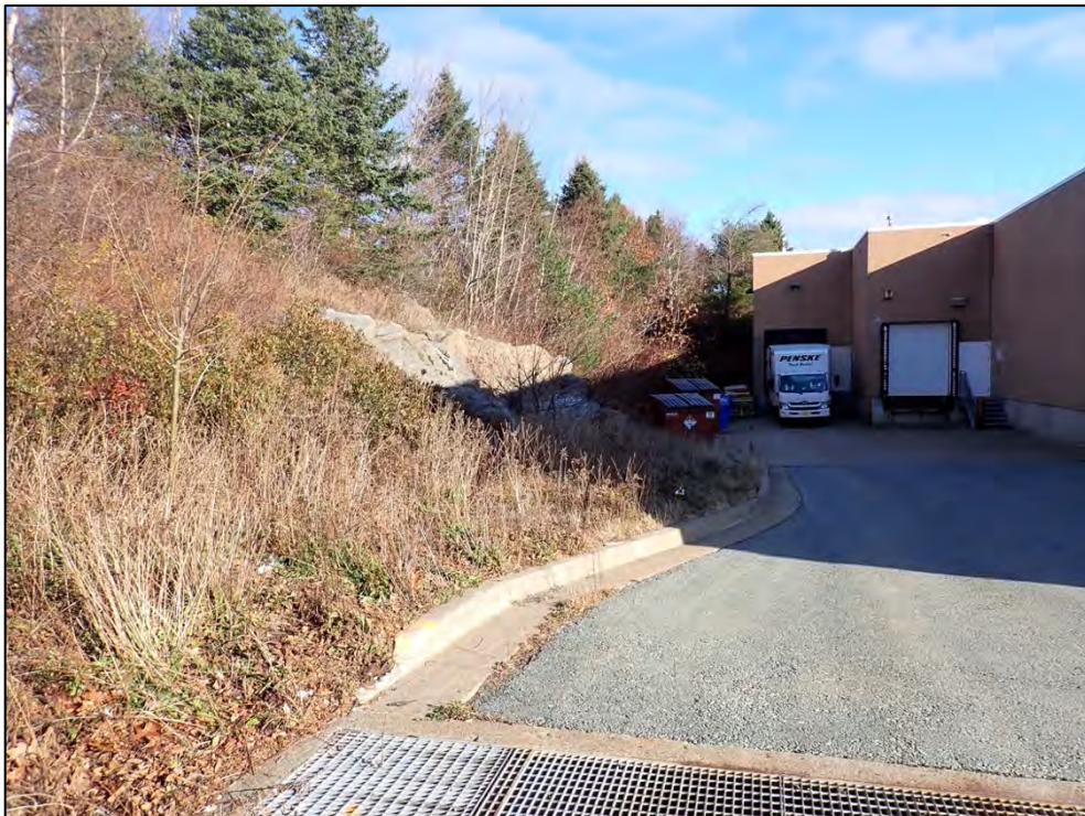
Plate 12: Looking northeast along the rear of the Chapters building showing the elevation change between the more natural grade at left and what has presumably been excavated out at the north edge of the study area.
