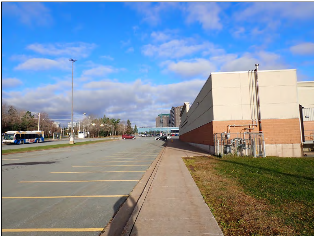
Plate 10: Looking north along the rear, or west side of the mall. The transit terminal can be seen to the left and natural gas connections can be seen on the right.
