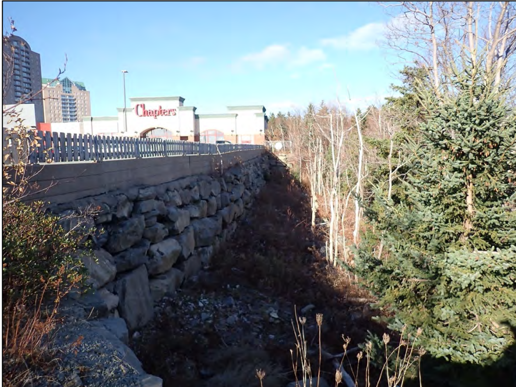
Plate 15: The treed area between Chapters' parking lot and Horizon Court looking north and showing the stone retaining wall and the sloping area.
