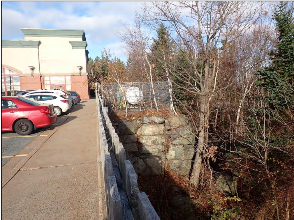
Plate 14: Looking north along the edge of the Chapters parking lot at a stone retaining wall.
