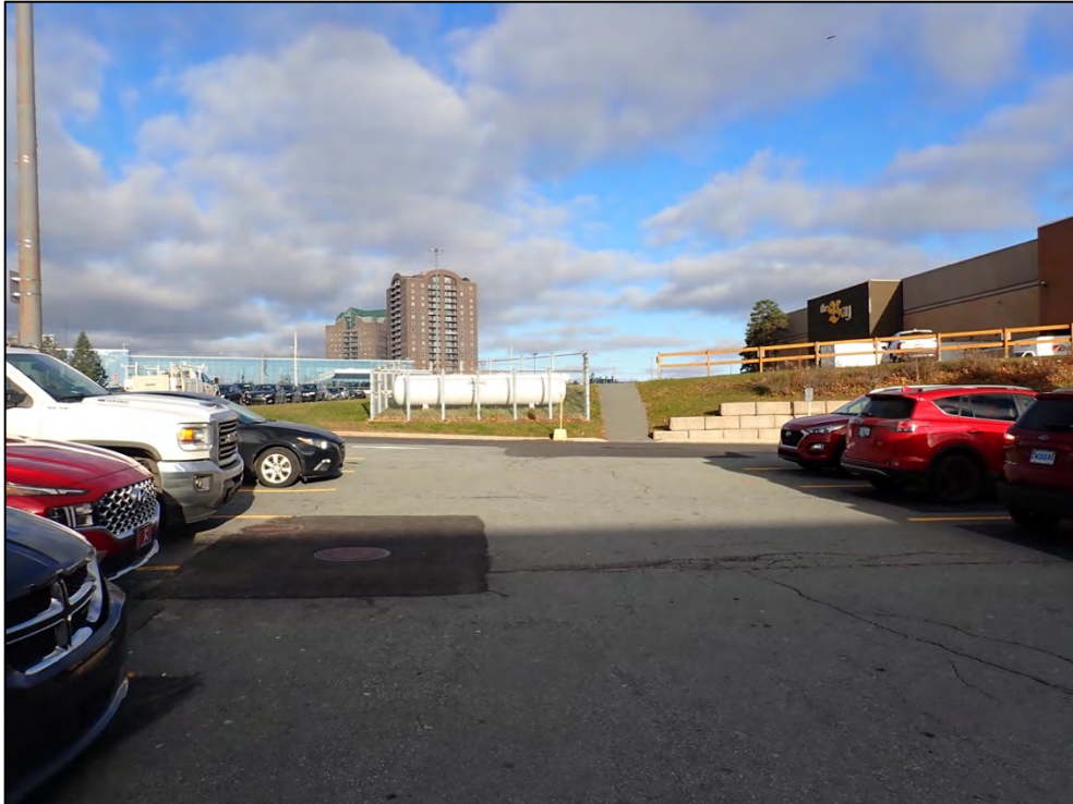
Plate 11: Looking north along the rear, or west, side of the mall at above-ground propane tanks. Note the elevation change between the parking lot in the foreground and that in the rear.
