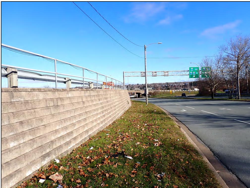
Plate 2: Looking east along the north side of Mic Mac Boulevard along the concrete retaining wall at the southeast end of the study area, which depict the level of infilling for the parking lot.
