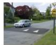
Speed Humps (reduce travel speed)
