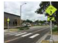
Flashing Lights (push button activated)
