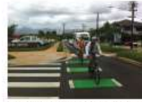
Painted Conflict Markings (carried through intersection)
