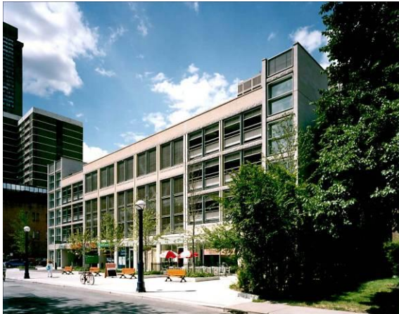
Charles Hayden parking garage in Toronto provides landscaping and pedestrian amenities to add to the street realm.
