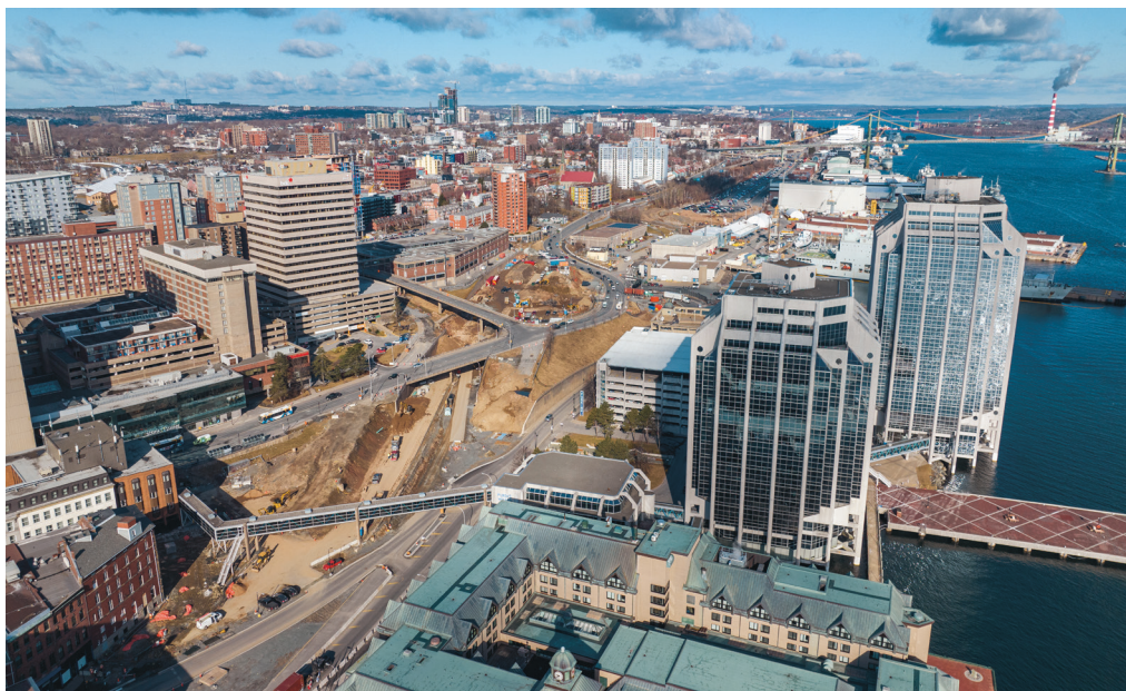
Existing site conditions as of March 2023
