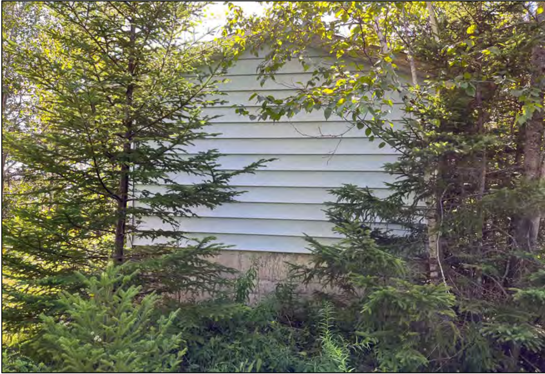
Plate 26: A small, potentially abandoned building with a concrete foundation in the woods to the east of the Halifax Exhibition Centre.
