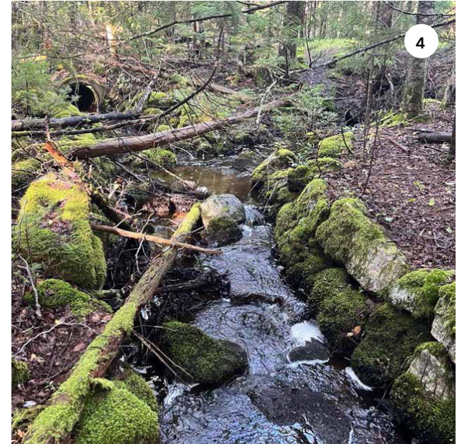
A culvert and stone-lined ditch, with some high and drier terrain around it.
