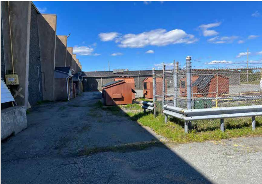
Plate 19: Propane tanks (enclosed in fencing to the right) and propane shut off switches on the building (yellow on left side), looking northwest.
