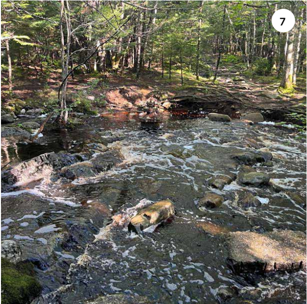
Cut granite blocks and parts of pipeline infrastructure were observable in the streambed.
