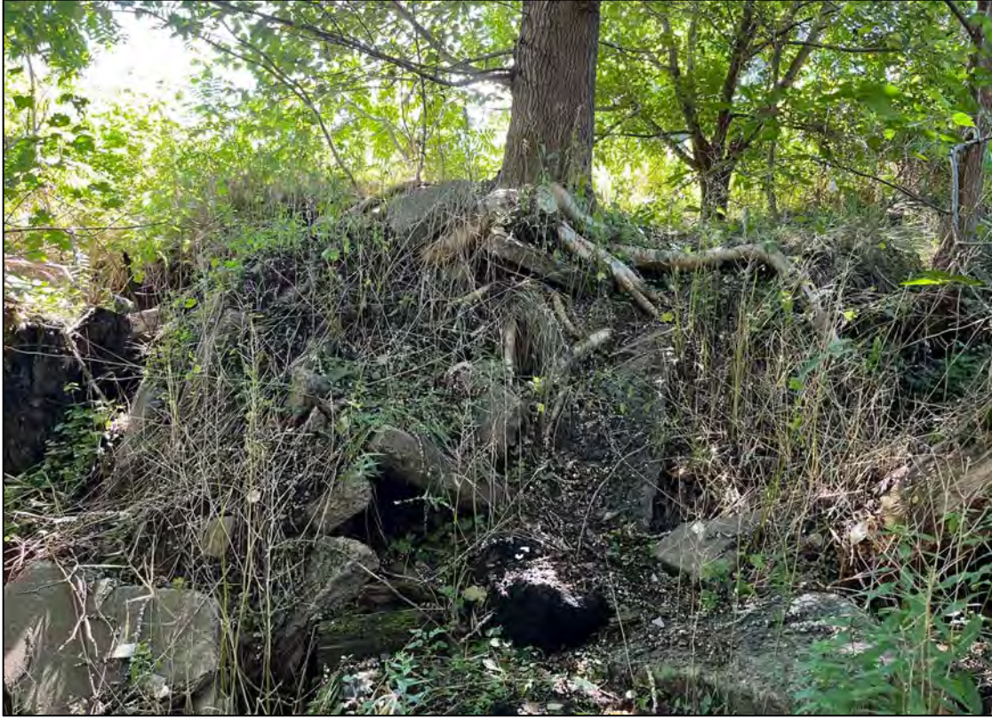
Plate 9: A mature tree growing on top of a pile of fill, including concrete blocks, looking west.
