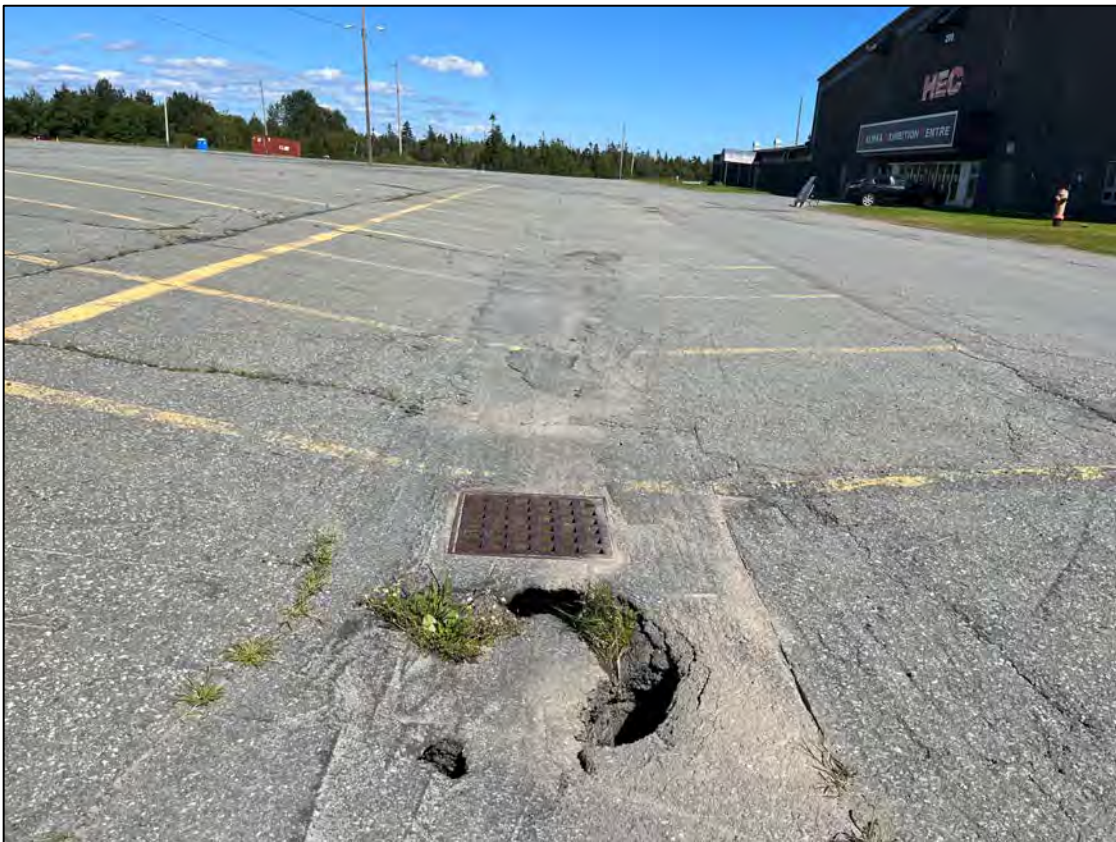
Plate 17: An existing stormwater drain and line in the parking lot in front of the Halifax Exhibition Centre, looking northeast.
