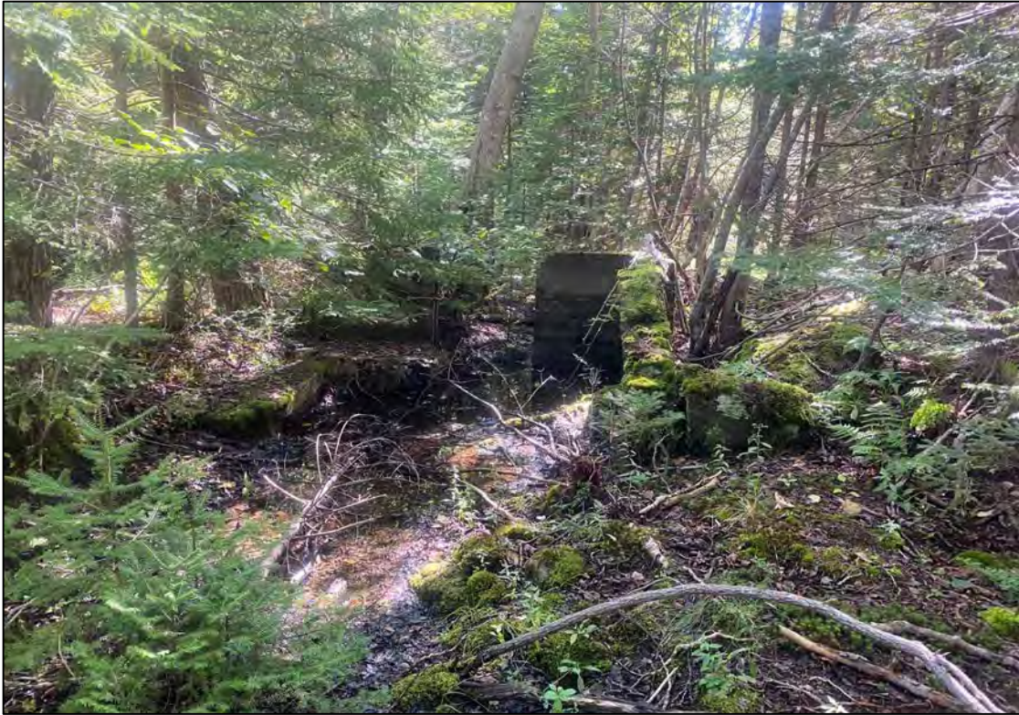
Plate 35: The remaining standing walls of the concrete foundation of Foundation_01, looking east.
