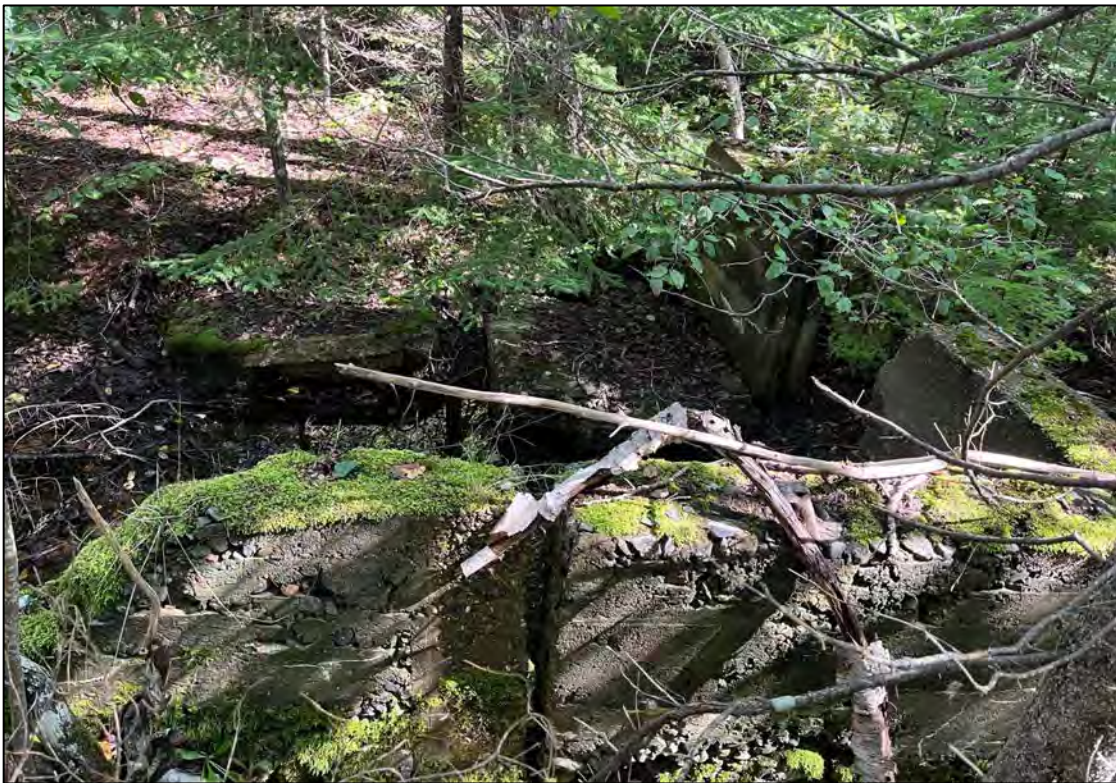
Plate 5: The concrete foundation (Foundation_01), looking north.
