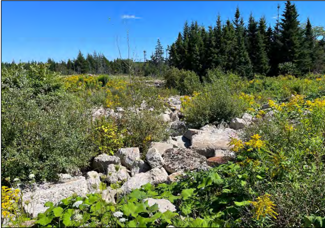
Plate 29: Large concrete block fill, with dense vegetation and goldenrod covering the fill, looking southeast.
