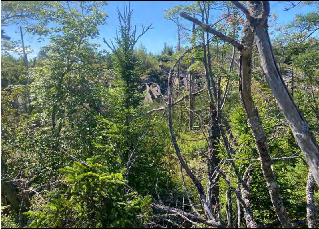
Plate 7: Large concrete blocks along the edge of the re-vegetating infilled slope, looking south.
