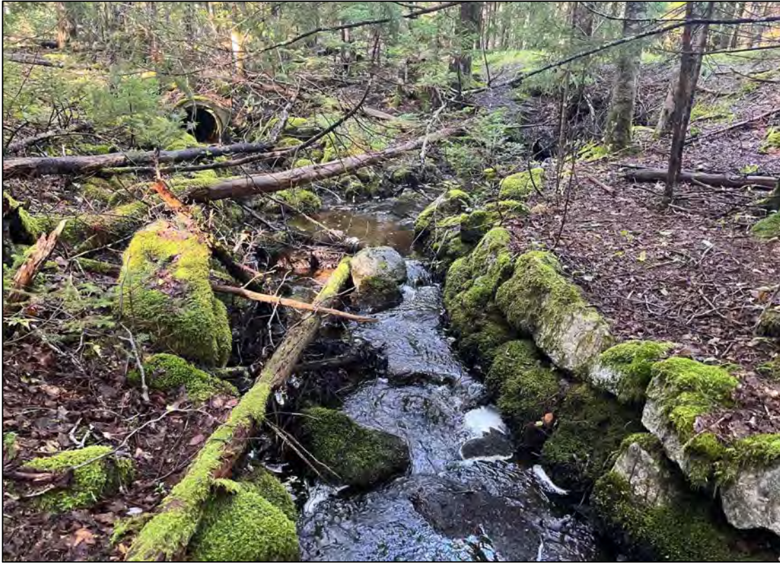
Plate 12: A stone-lined ditch leading from a culvert to the brook, along the gravel trail (right), facing southwest.
