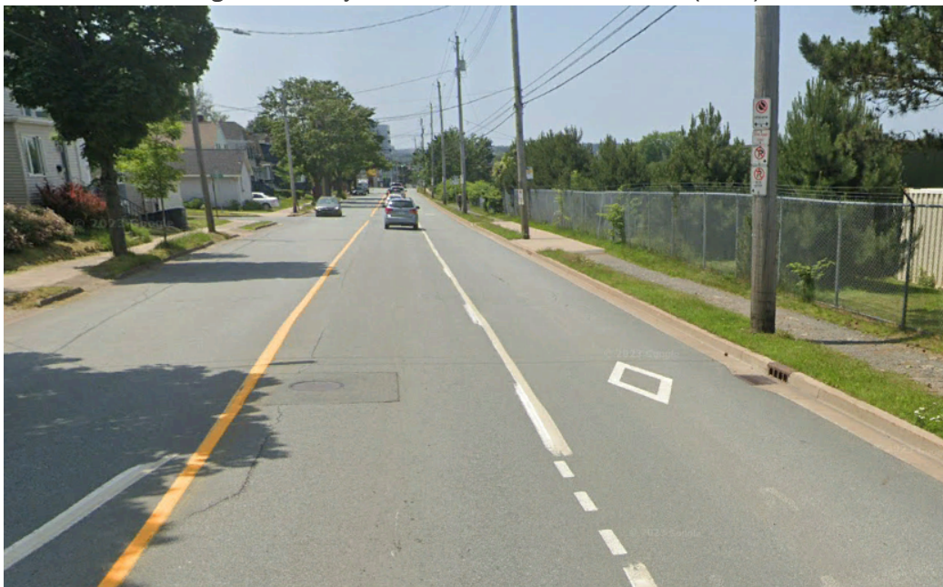
Figure 3-50: Bayers Road Pilot Outbound Bus Lane (2023)
