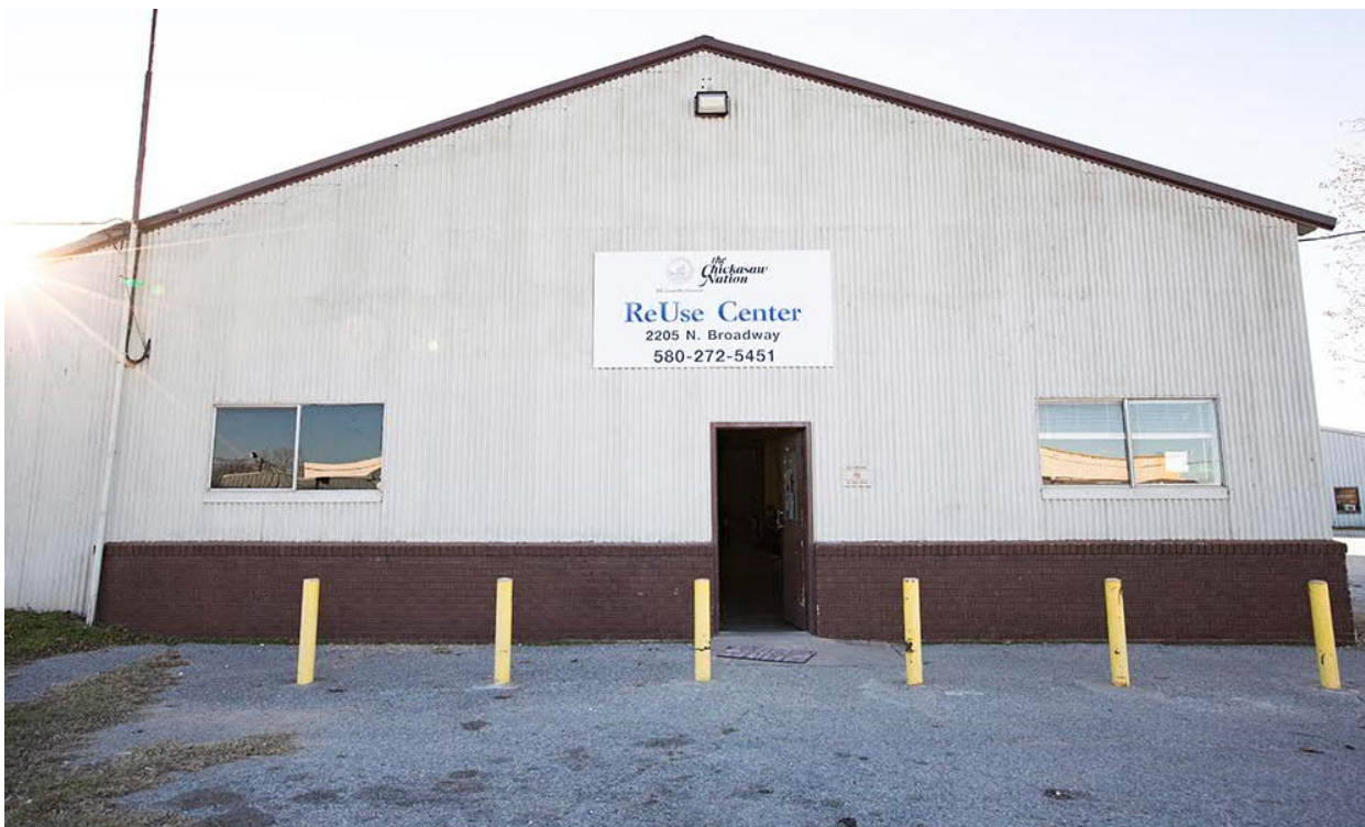
Photo 10: Typical Pre-engineered Building - ReUSE Centre Building, Chikasa Nation, Oklahoma
