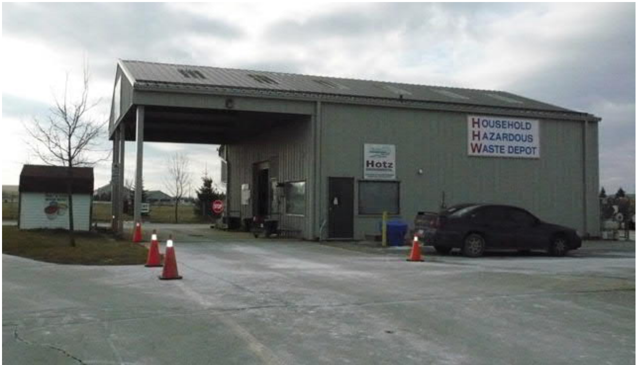
Photo 1: Pre-Engineered Steel Structure: Halton, Ontario HHW Depot
