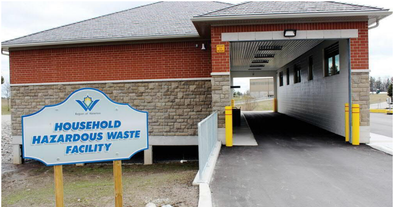
Photo 2: Masonry Construction Structure: Region of Waterloo, Ontario HHW Facility
