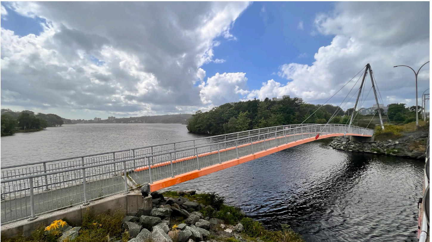
Active Transportation bridge crossing Lake Banook
