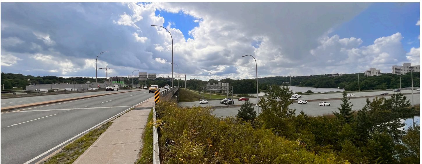
View of the Braemar overpass from Waverley Road
