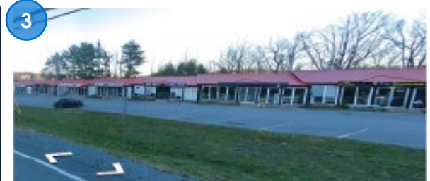
Strip mall containing retail and services, 12 Esquire Lane
