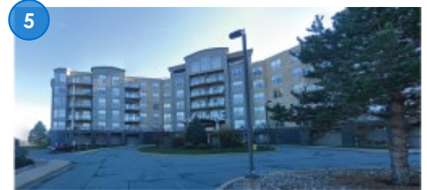
Six-storey multi-unit residential, 36 Southgate Drive
