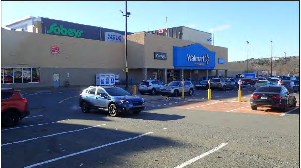
Plate 10: Walmart storefront and parking lot, facing southwest.
