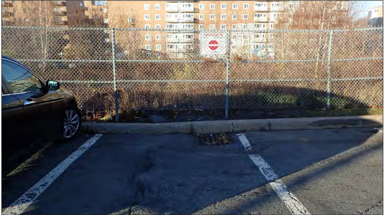
Plate 5: Catch basin at the west extent of the study area, facing west.
