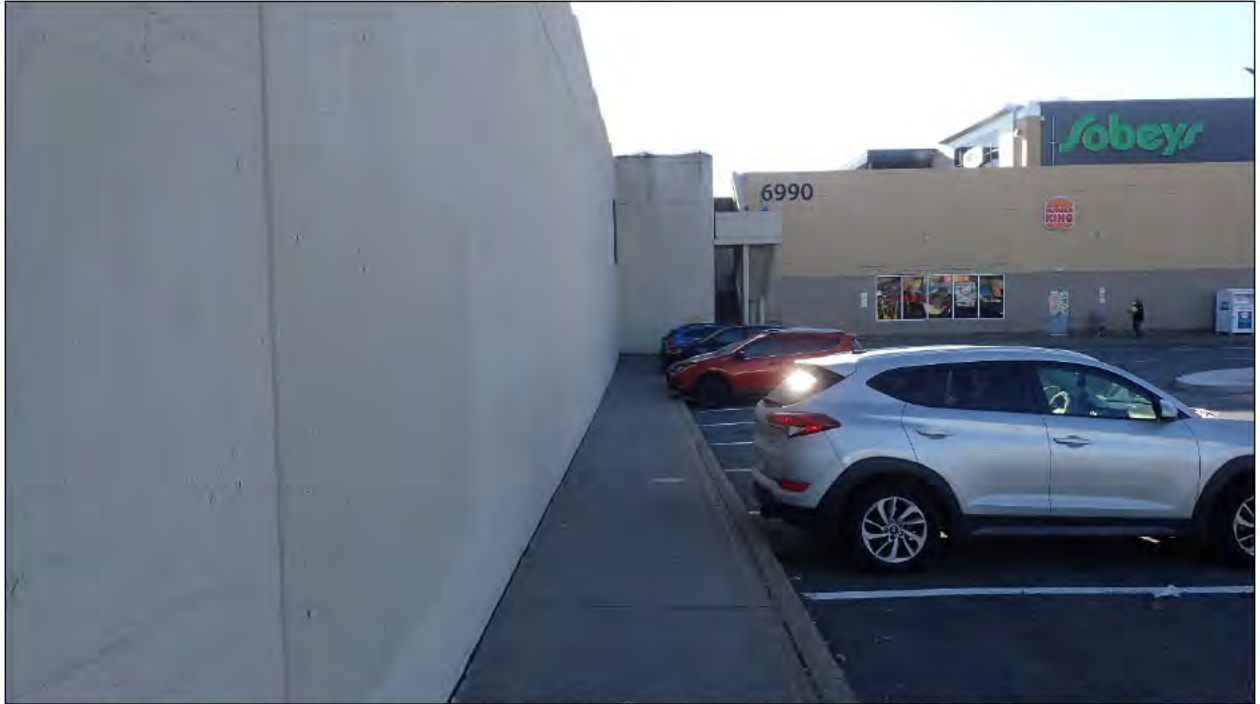
Plate 11: Concrete retaining wall (left) at the east end of the Walmart parking lot, facing southeast.
