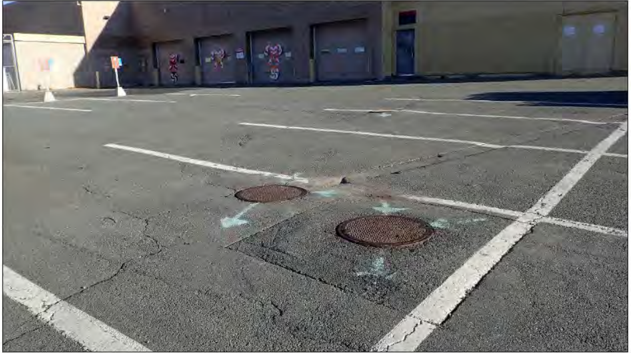
Plate 7: Manholes in the parking area with the Walmart trucking bays in the background, facing northeast.
