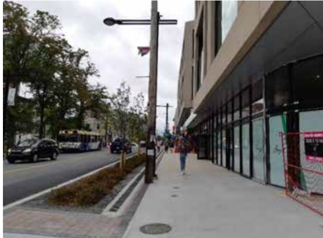
The recently constructed Doyle Block on Spring Garden Road achieves a wider pedestrian realm through ground-level building setbacks
