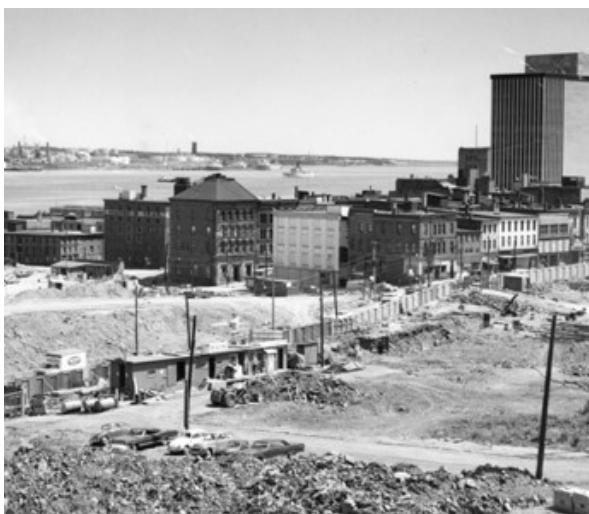
Scotia Square and Cogswell Interchange construction (c. late 1960s)
