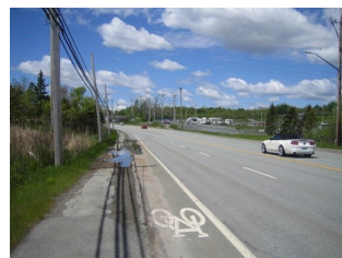
Photo 5 - Looking west on Main Street from site driveway 130 m west of Westphal Way.
