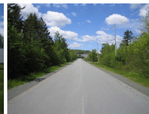
Photo 7 - Looking west on Giberson Drive towards Broom Road.
