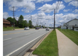
Photo 2 - Looking east on Main Street towards Cherry Brook Road from Wilfred Jackson Way.
